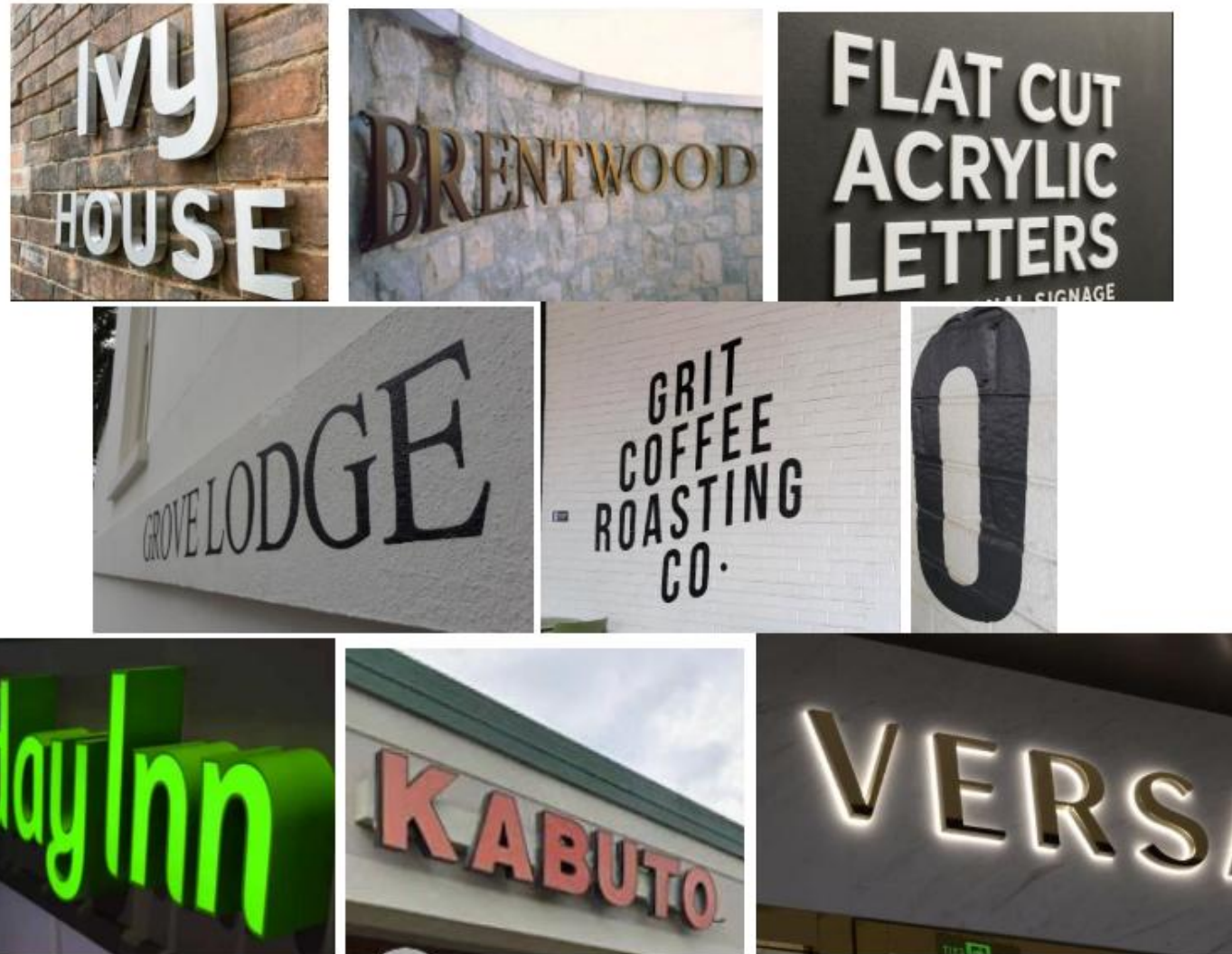
Various individual letter signs: Top: individual cut out letters of varying dimensions, left and right direct-mounted; middle pin-mounted. Middle: painted letters (left) and vinyl letter sign (middle) with vinyl letter detail (right). Bottom: internally illuminated, face lit channel letters (left), channel letters on raceway (middle), halo-lit channel letters (right).
